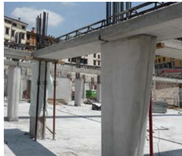
Travi PREM a2 Pilastrini in opera PREM a2 Beams Cast in situ Columns
